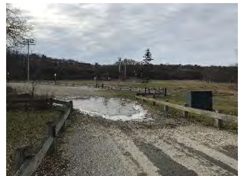
The main parking area with drainage issues
