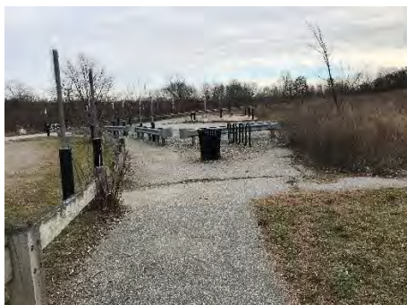
Cracked and uneven pathways
