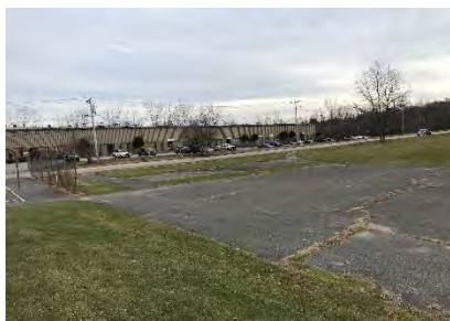
The open pavement area
