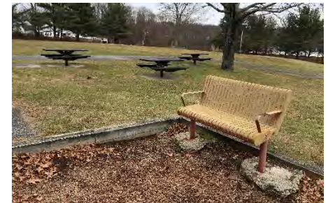
Site bench with exposed foundations
