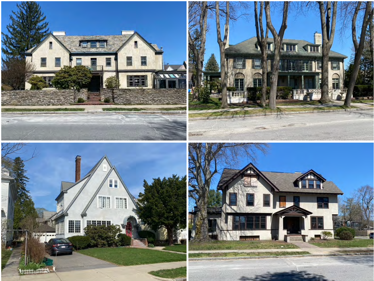
Examples of buildings with stucco exterior walls in Worcester’s local historic districts.
