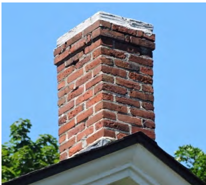
Maintenance of chimneys is important, especially when they are not highly visible and are hard to reach. The chimney at left has open joints which let water enter the brickwork, causing deterioration. The flashing in the chimney at center is critical in protecting the roof from water penetration. A metal chimney cap has been installed on the chimney at right to prevent sparks from threatening the roof.
