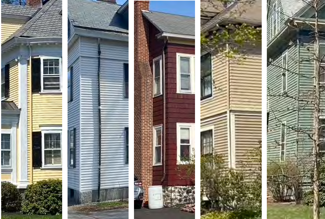
Gutters and downspouts can be designed in response to building character. Many buildings in Worcester’s local historic districts were built without gutters, and some have had them later installed. The two buildings at left above have built-in gutters in conjunction with slate roofs. The gutter installation at center used the eave extension to position the downspout to the side of the front elevation. The two examples at right painted their downspouts to match the exterior wall colors to reduce their visibility.
