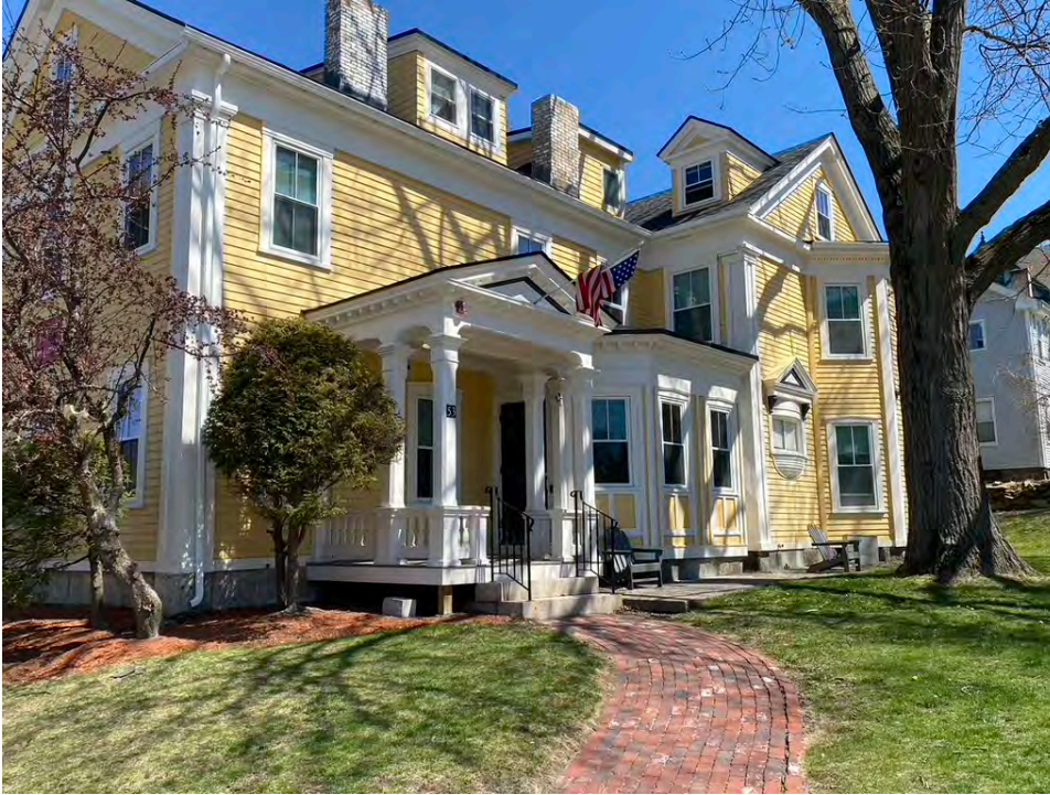
Most residences in Worcester's historic neighborhoods are of wood frame construction with wood siding, features, and details.
