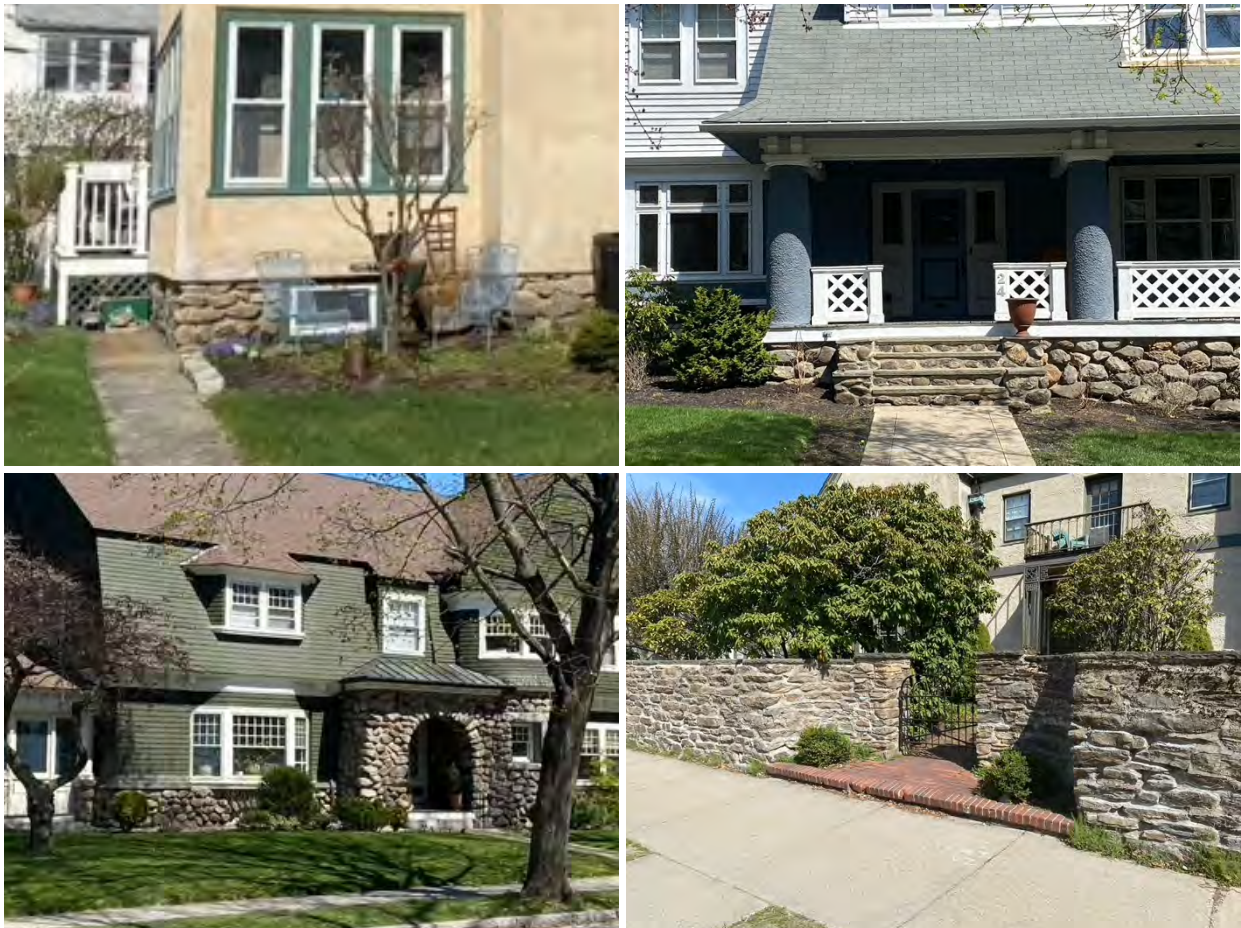
Uses of stone within Worcester's local historic districts – as foundation walls in the upper photos, as a foundation wall and decorative entranceway lower left, and as an exterior wall lower right.
