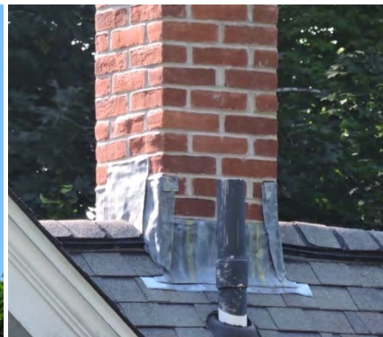
Maintenance of chimneys is important, especially when they are not highly visible and are hard to reach. The chimney at left has open joints which let water enter the brickwork, causing deterioration. The flashing in the chimney at center is critical in protecting the roof from water penetration. A metal chimney cap has been installed on the chimney at right to prevent sparks from threatening the roof.
