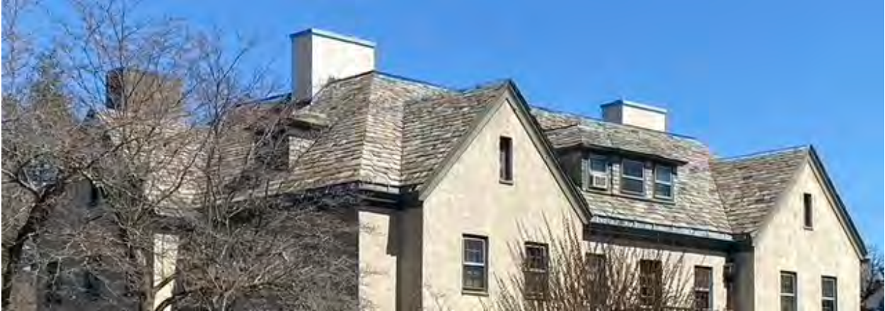
Preserved slate roof in the Elm Park Neighborhood, remaining in good condition after over one hundred years.
