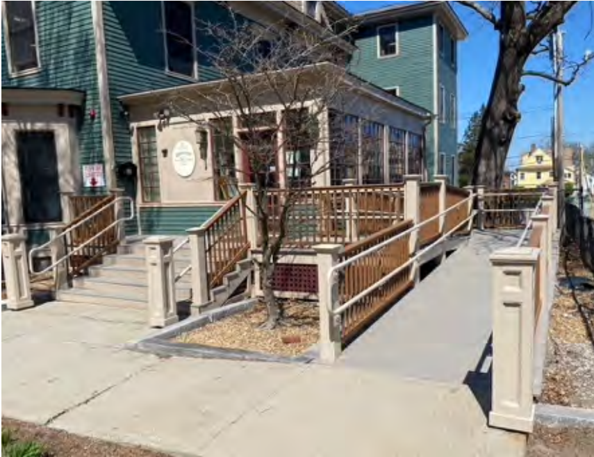
Fully compliant ADA accessible ramp installed adjacent to a historic vestibule entrance for a historic residence adapted to a family resource center in the Elm Park Neighborhood Local Historic District.
