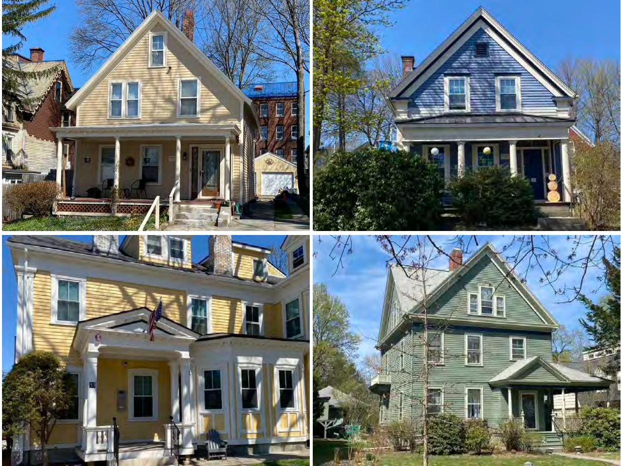
Representative buildings within Worcester’s local historic districts with preserved original, authentic wood windows protected by exterior storm windows.
