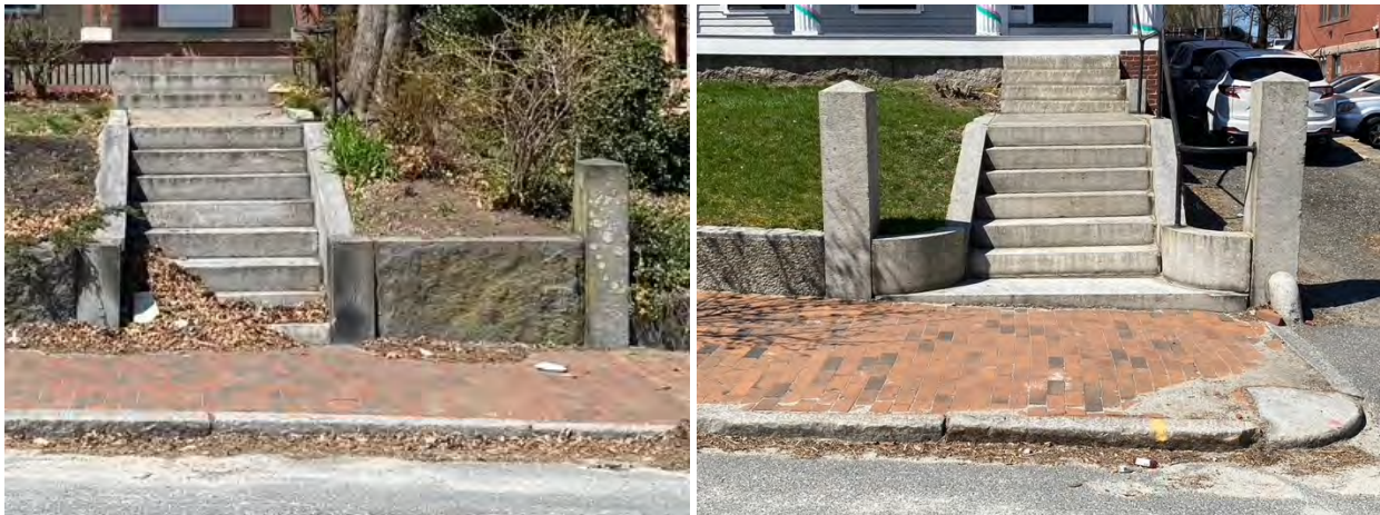
Granite street curbs, retaining walls, posts, and front steps are common throughout the Crown Hill and Elm Park Neighborhood Local Historic Districts and should be preserved and maintained. In these two locations, brick sidewalk paving remains as well.
