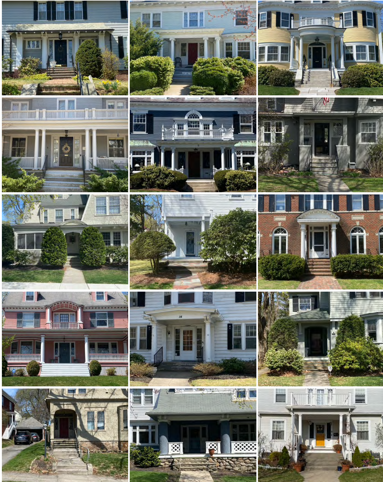
Sampling of the variety of historic entrances within Worcester’s local historic districts. Each is designed as a featured element, contributing to the architectural character of its building. Each provides a welcoming experience, with steps up to the first-floor level, a sheltering overhang, and fine detailing. Most feature sidelights beside the front door for a more spacious and light-filled interior/ exterior experience.
