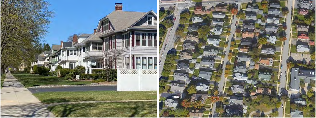
In the Elm Street Neighborhood’s West Side Realty area above, buildings vary in the details of their forms, but are regular in their overall massing, are close together, are wide and deep, and are uniform in their setbacks.
