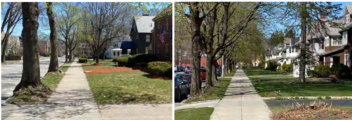
Concrete sidewalks are most common within the local historic districts, many of which are original.
