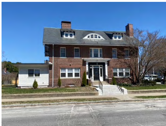
Eclectic , 2-story brick residence at 66 William Street built in 1909 with a symmetrical façade, exterior chimney, and deep open eaves.
