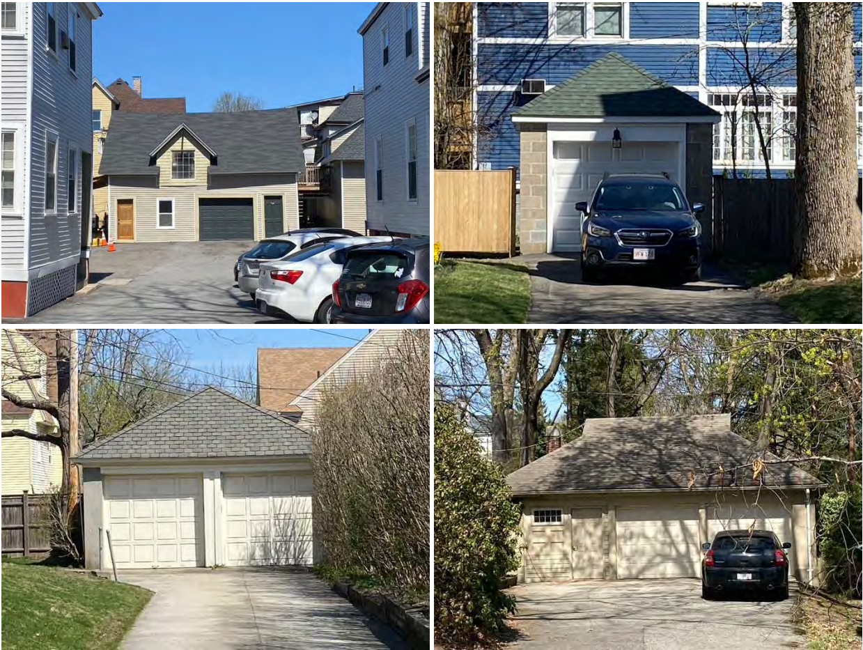
Existing garages in Worcester’s local historic districts tend to be either converted carriage houses (top left) or small one- or two-car garages of the type built in the early 20 th century when car ownership was just beginning. These historic garages should be preserved, and new garages should draw design inspiration from them.
