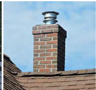
Maintenance of chimneys is important, especially when they are not highly visible and are hard to reach. The chimney at left has open joints which let water enter the brickwork, causing deterioration. The flashing in the chimney at center is critical in protecting the roof from water penetration. A metal chimney cap has been installed on the chimney at right to prevent sparks from threatening the roof.
