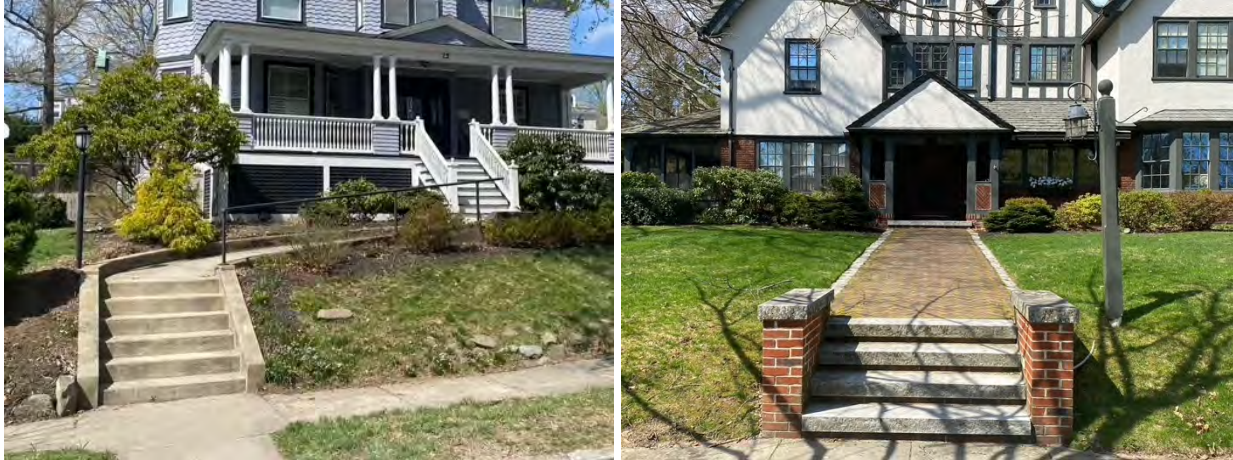
Concrete front steps (left) are common throughout the historic districts and in some cases probably replaced earlier granite steps. The granite and bricks steps, walls, and walk at right are customized to the character of the Tudor residence to which they belong.
