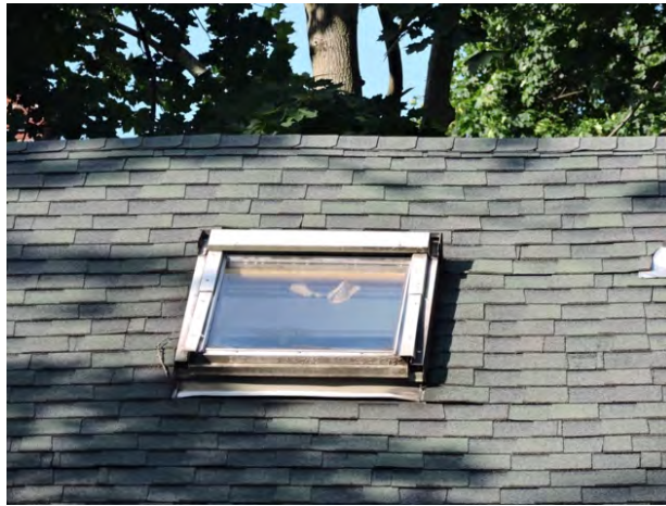
Skylights may be installed on side and rear elevations. They may be operable but should be low profile, as the one shown here.
