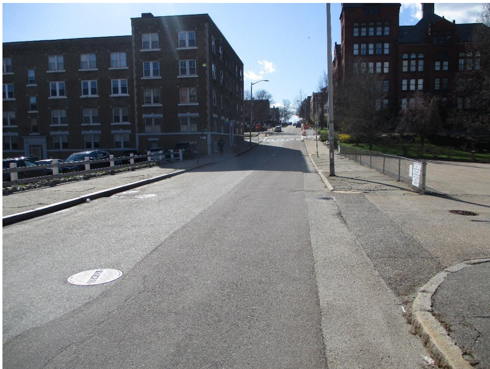
Facing West on Chatham Street
