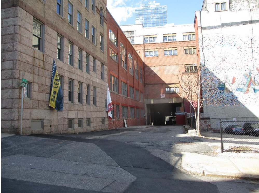
View of Chase Court Traversing Beneath Building on Parcel 1
