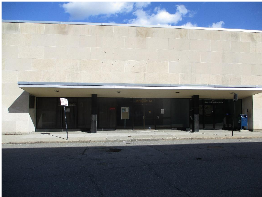
West Side of the Building on Parcel 1
